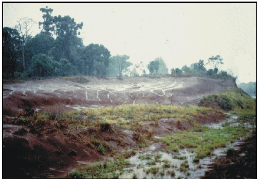
**Fig. 5-2:** Rill erosion and deposition at the foot of the slope after road construction. San Pedro, Misiones (Photo: M.F.Rau, 2001).
