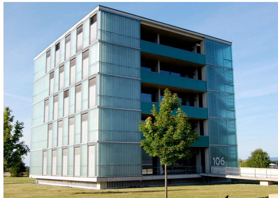
Figure 4.3: Building 106 on the Freiburg computer science campus.
