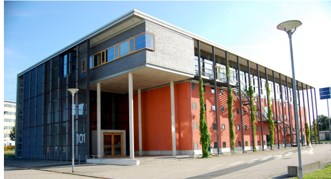
Figure 4.7: Building 101 on the Freiburg computer science campus.
