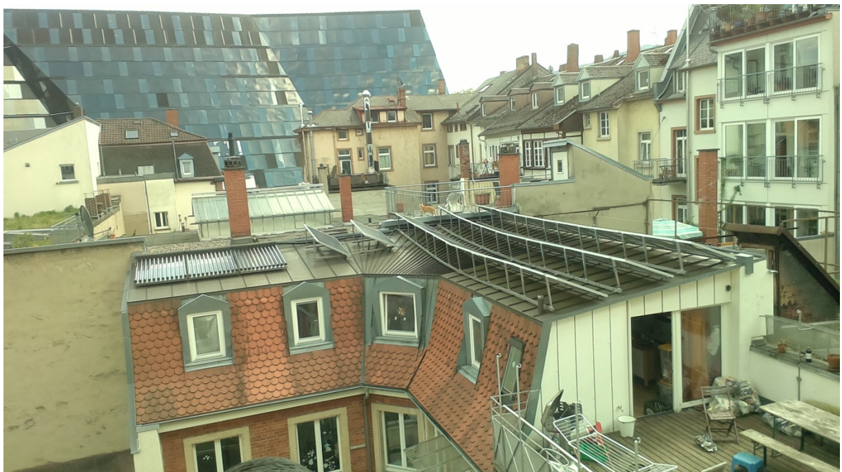
Photo 4.3: Combination of PV on the roof and Cogeneration of Heat and Power (CHP) at a dwelling in the city centre of Freiburg.
